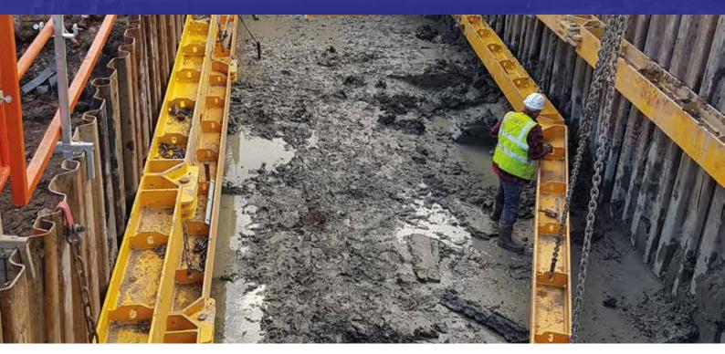
Meever series Brace is a modular system designed & engineered to maintain excavation integrity, it allows flexibility on site and saves time and money. Most importantly it provides a safe working environment.
